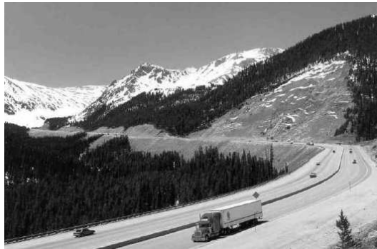
Figure 4.5: Interstate 70 in Colorado USA. 5–7% 10 miles long downhill slope with downhill truck speed warning system. With permission from: Oregon Department of Transportation Traffic Engineering & Operations, ITS Unit.
